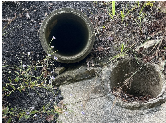
Figure 16: Failed headwall.
